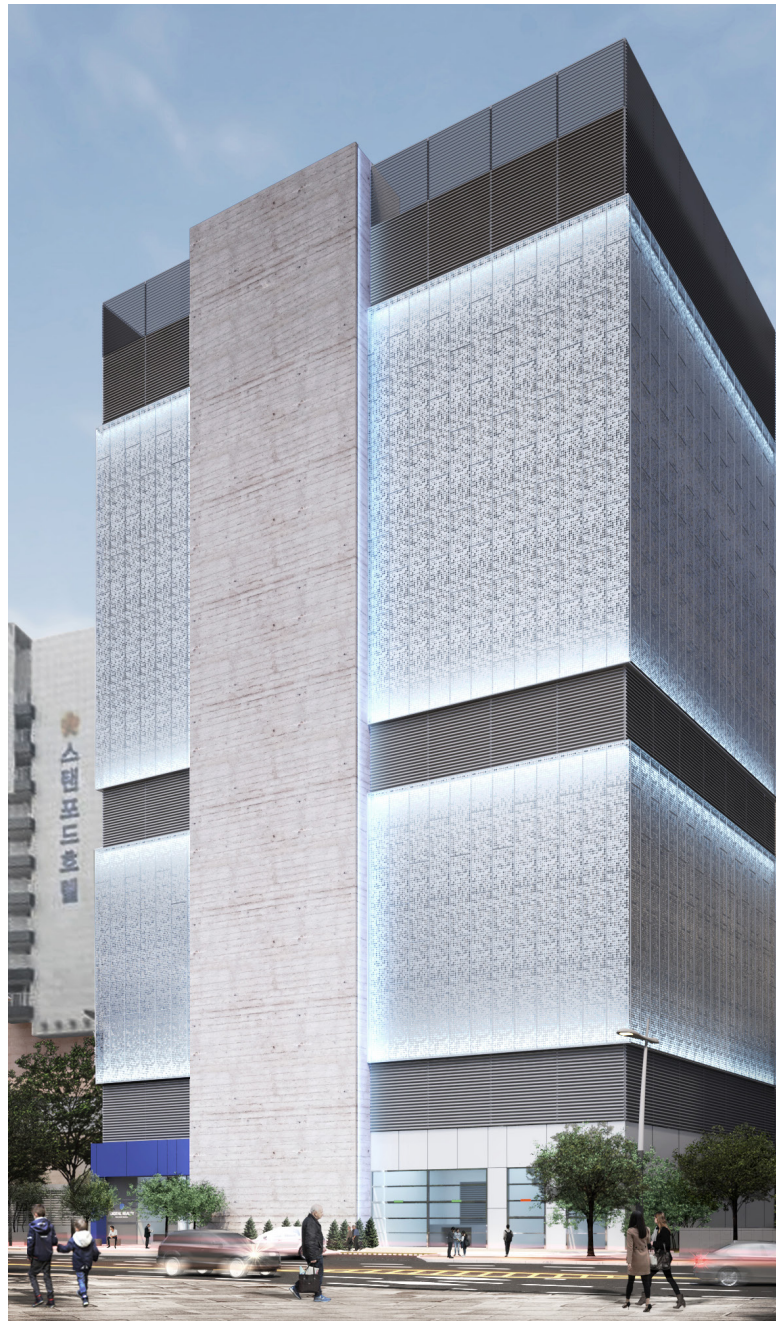
ICN10 data center, Seoul, South Korea
