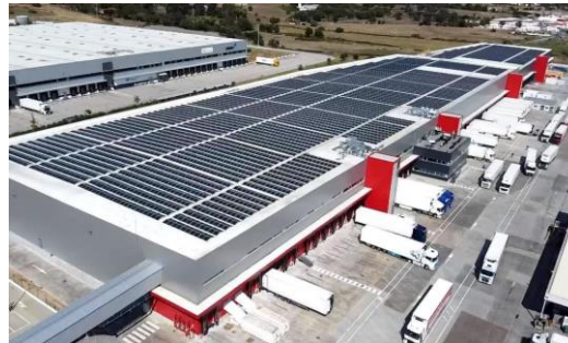
Sonae Completed September 2020
