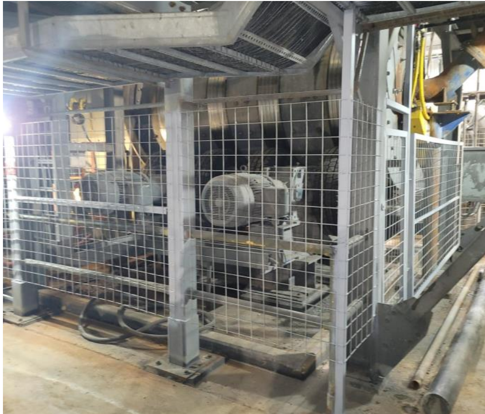
Primary Ball Mill: Guarding Installed
