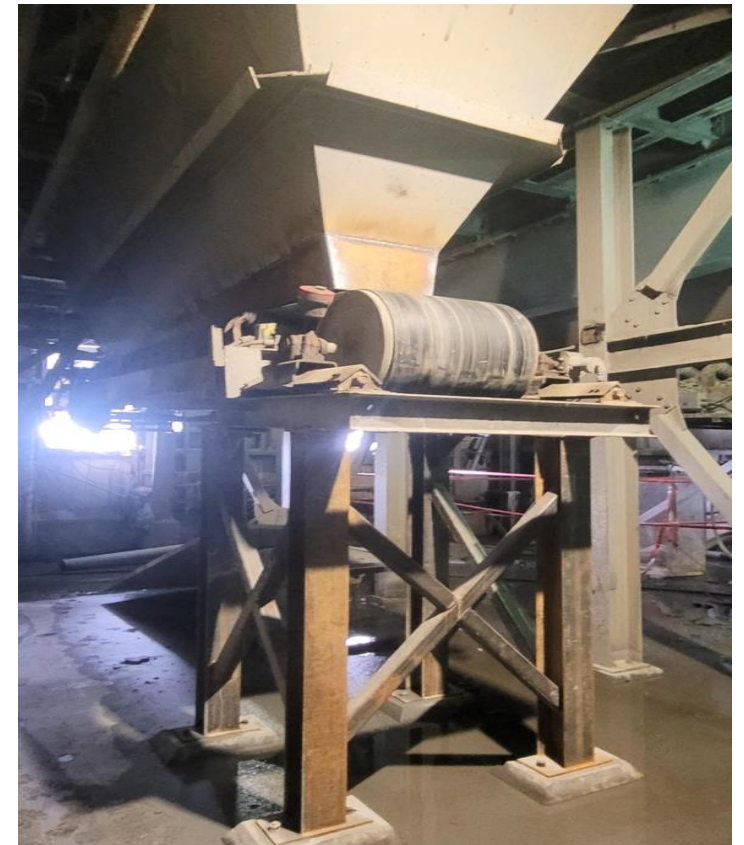
Tailings Discharge Chute
