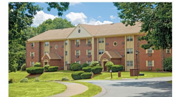
Wexford Village 264 Units – Worcester, MA
