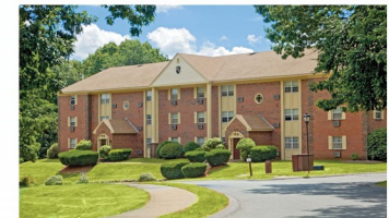
Wexford Village 264 Units – Worcester, MA
