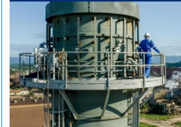
Clarendon CHP Plant
