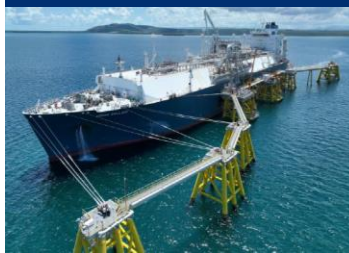
Old Harbour Terminal
