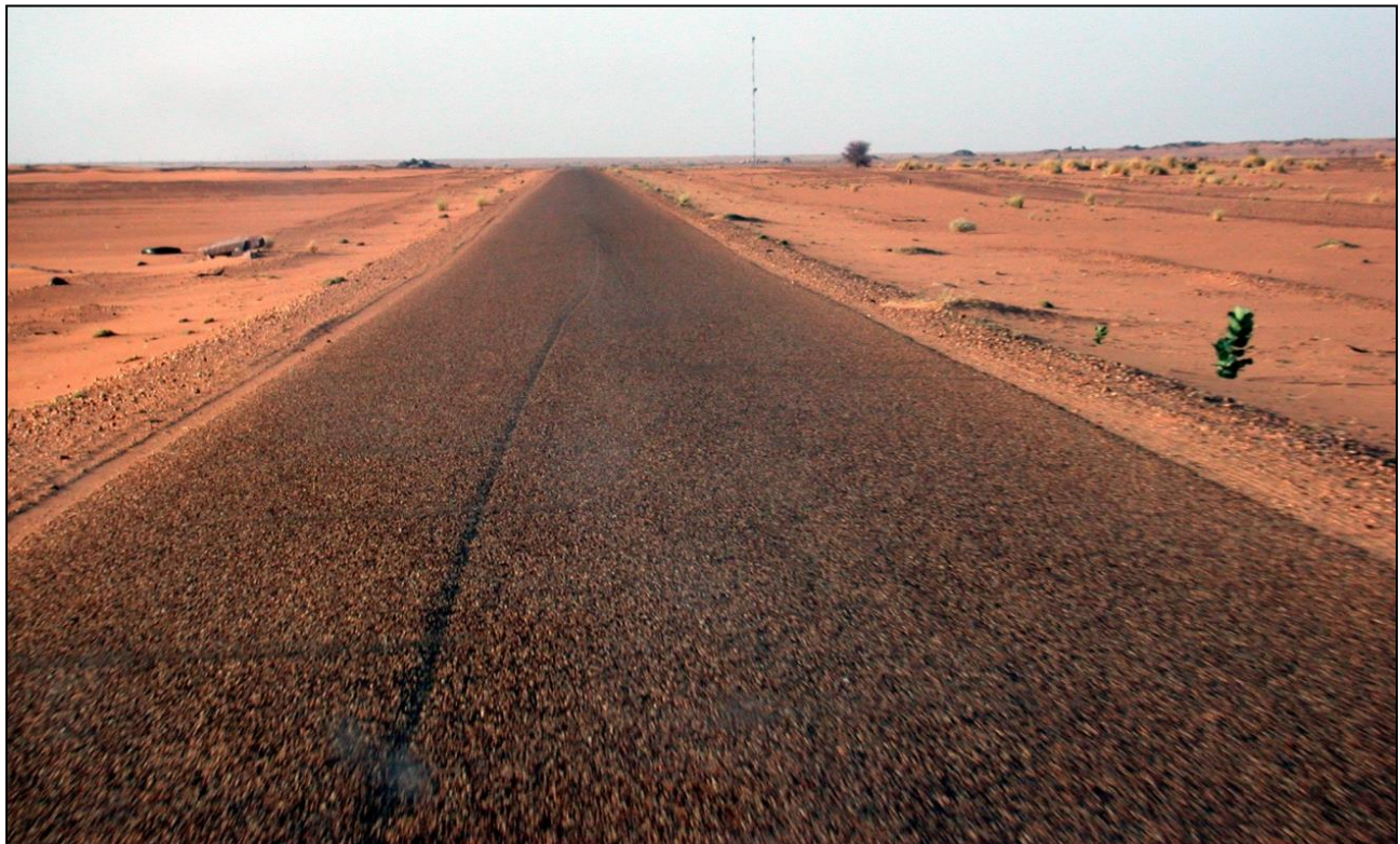
Figure 5-1: Road N25, just north of Agadez Source: GAFC
