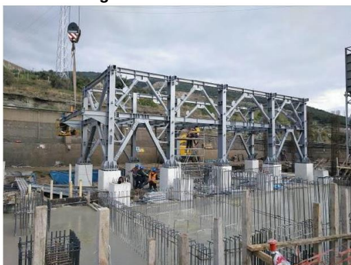
Settling Chamber Construction
