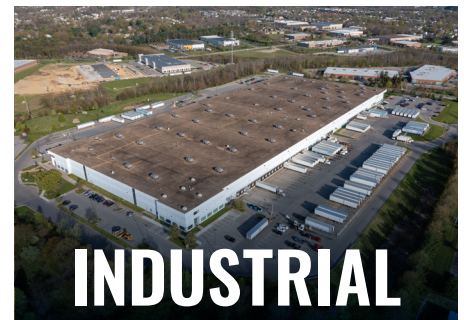
Warrendale, Pennsylvania 430,613 Interior Square Feet
