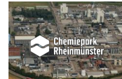
Acquired additional latex binder assets at Rheinmünster, Germany Site
