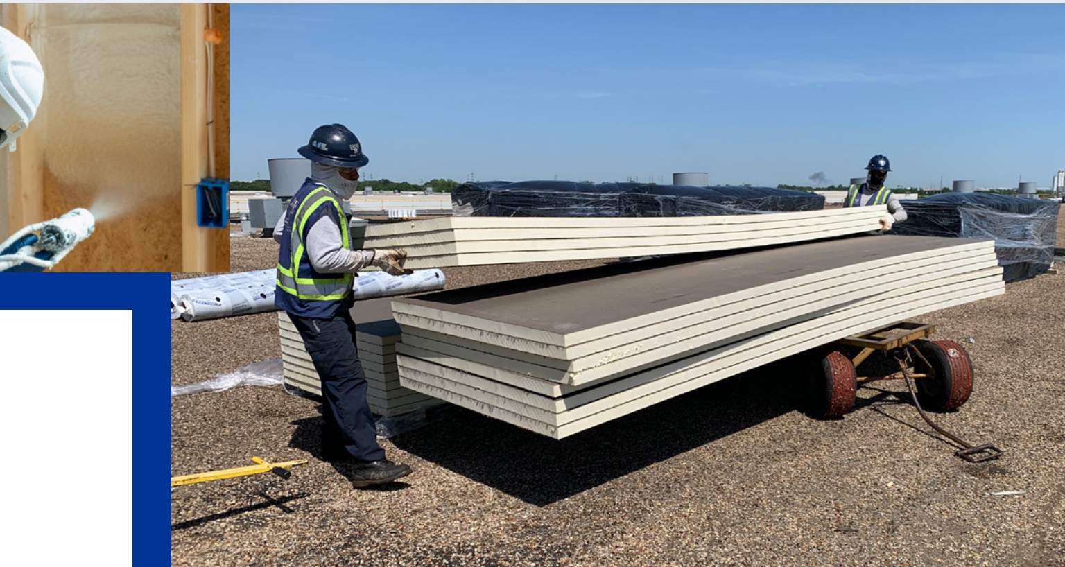
Carlisle SynTec's new 12' polyiso reduces loading time, fastener use, and installation labor
